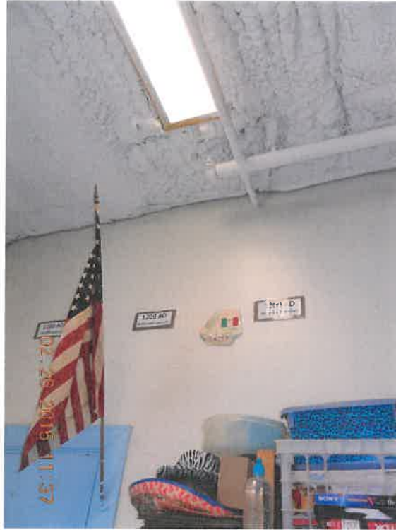
Room 302 - 303 - foam insulation on roof deck. Not able to inspect.
