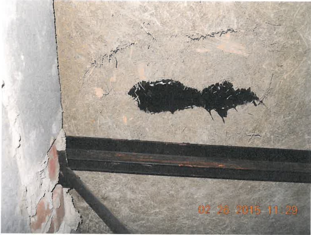
Girl's bathroom - damaged Tectum roof deck
