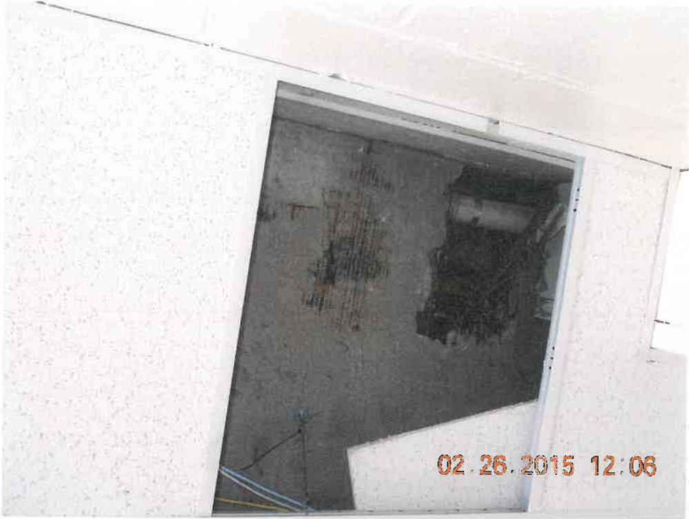
Room 224 - old ceiling metal lath and plaster. Roof not observable.
