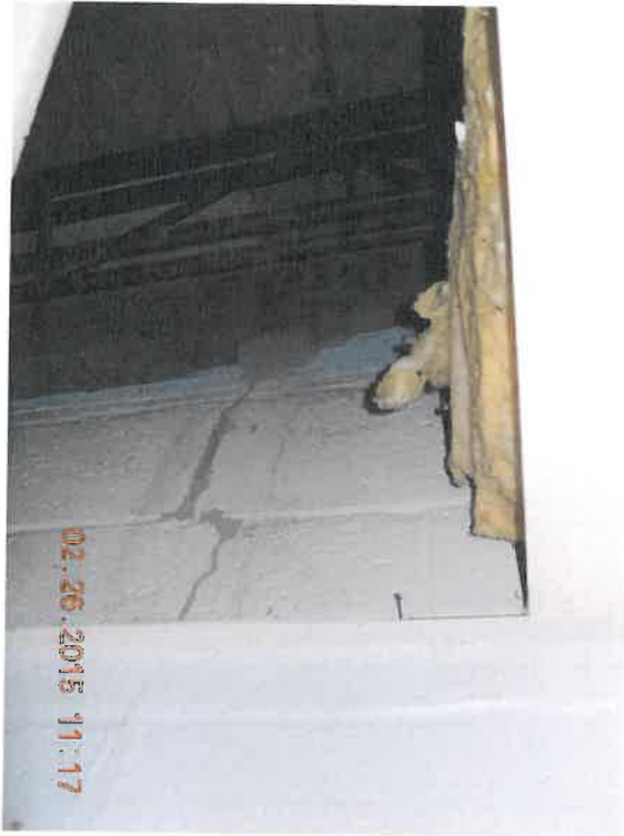
Old crack repair
