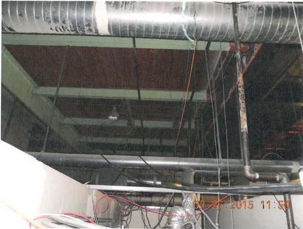
Above library - wood deck and steel beams
