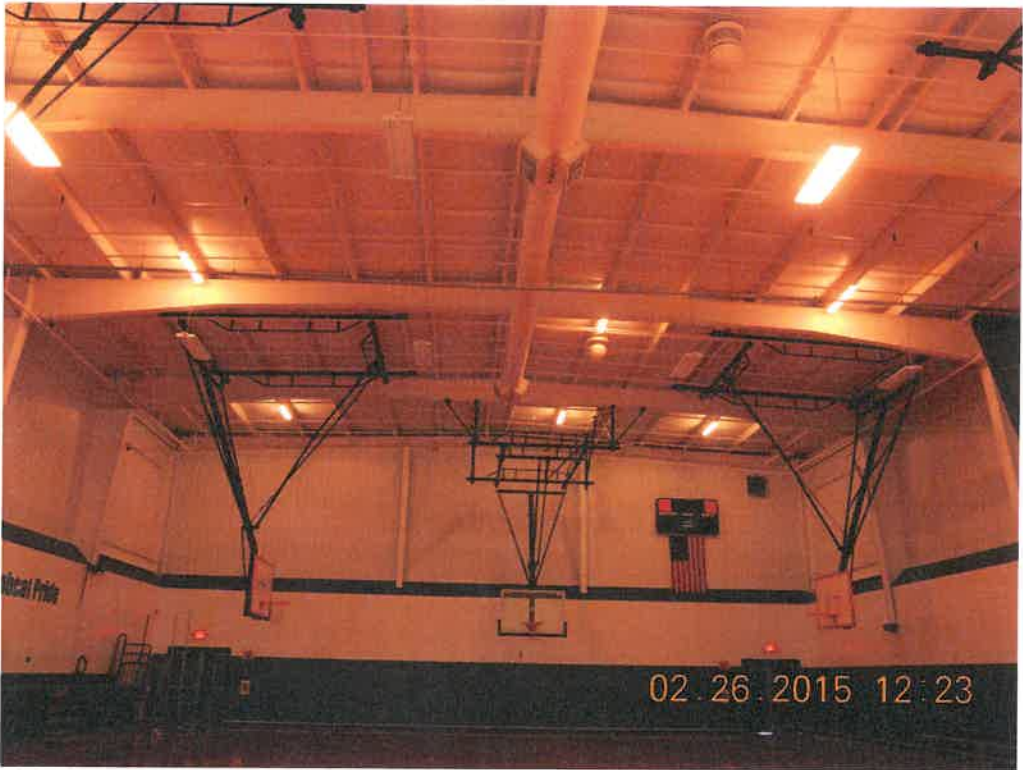
Gym - no damage found
